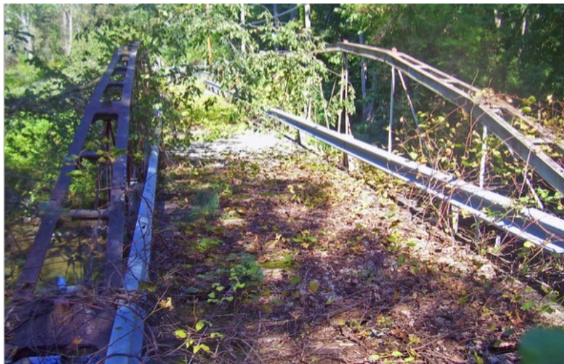
Recent Photograph of abandoned in place bridge.
