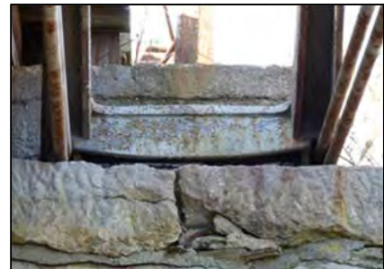
Figure 7 Examples of inappropriate repairs: (a) Retainer plate on top chord; (b) Hairline crack (from holes for guardrail support) made potentially worse with more steel patch holes; (c) End of chord encased in concrete.
