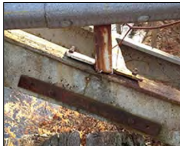
Figure 7 Examples of inappropriate repairs: (a) Retainer plate on top chord; (b) Hairline crack (from holes for guardrail support) made potentially worse with more steel patch holes; (c) End of chord encased in concrete.
