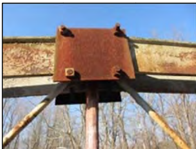
Figure 7 Examples of inappropriate repairs: (a) Retainer plate on top chord; (b) Hairline crack (from holes for guardrail support) made potentially worse with more steel patch holes; (c) End of chord encased in concrete.
