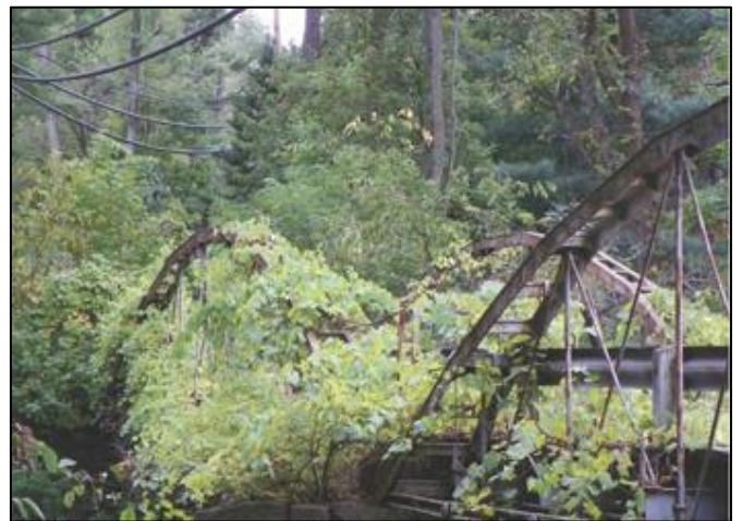
Figure 6. Shaw Bridge. Photo by Rick Ehrenberg 2010
