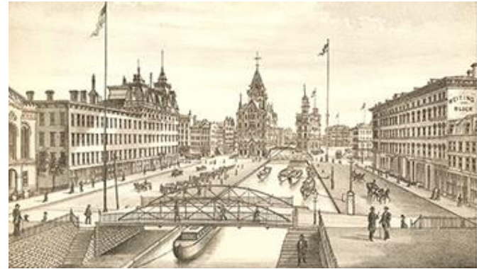
Figure 3. Lithograph of Whipple's Bowstring Bridge in Syracuse NY, one of hundreds built over the Enlarged Erie Canal.
